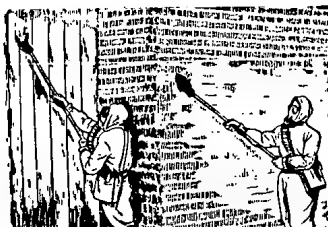
Decontamination of Walls with the Calcium Chloride Paste.
